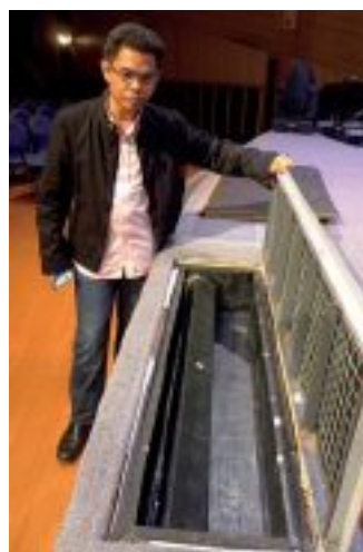
Church consultant Erwin Balague reveals one of the four hidden K-Array KP102 speakers that serve as stage monitors
